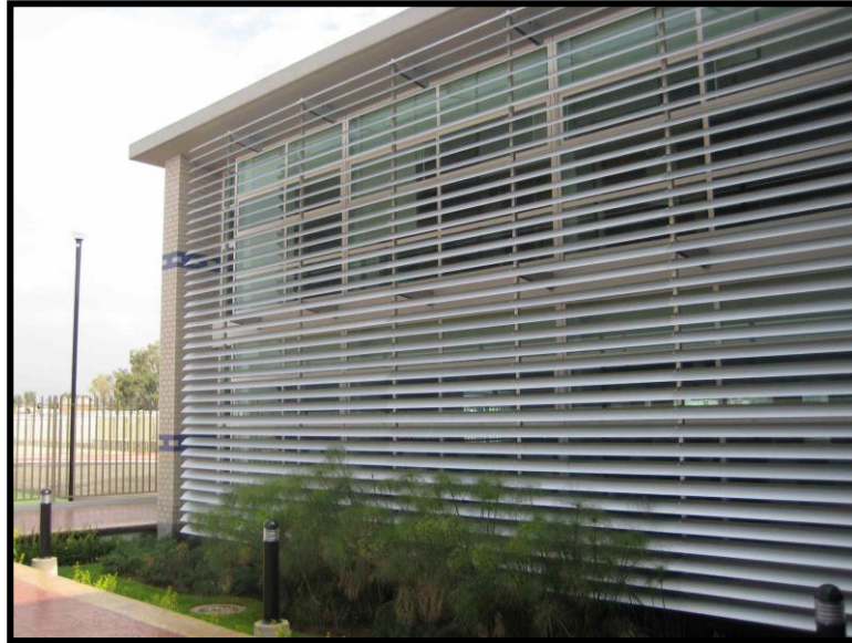
Figure 2.10: Typical glazing panel with sun louvers
