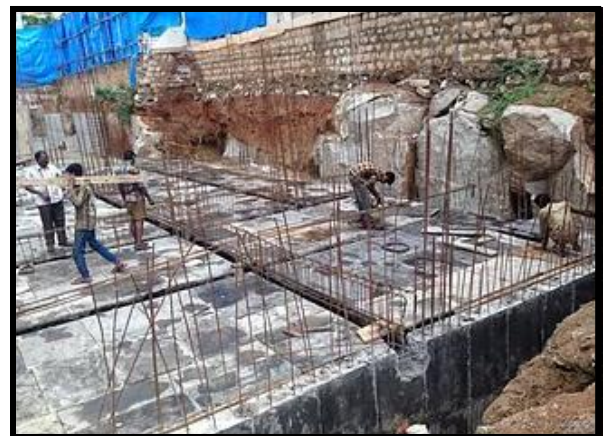
Figure 0.4: Steel and RCC structure
