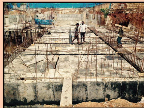
Steel and RCC structure
