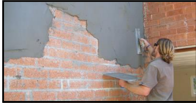
Figure 2.4: Bricks with concrete plastering
