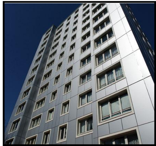
Figure 2.14: Building etalbond rain screen panel
