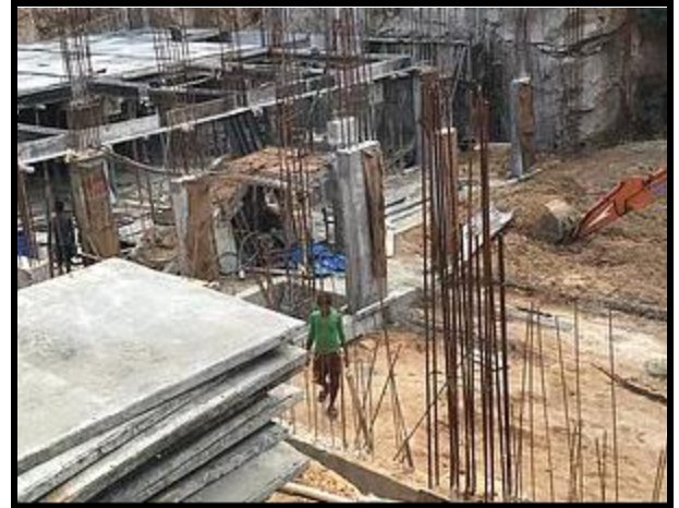
Figure 0.5: Metal shuttering sheets for formwork
